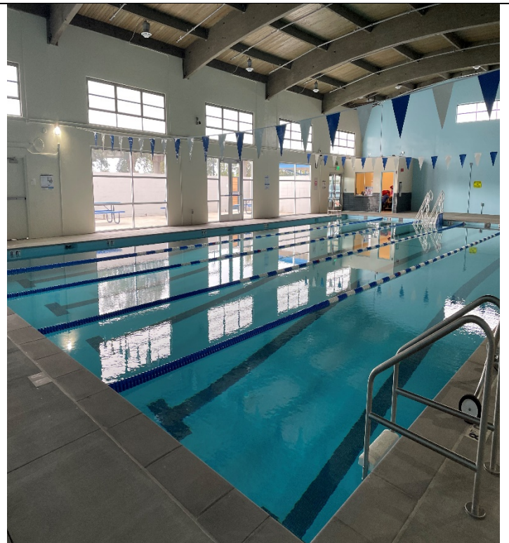
COMPLETED POOL ROOM
